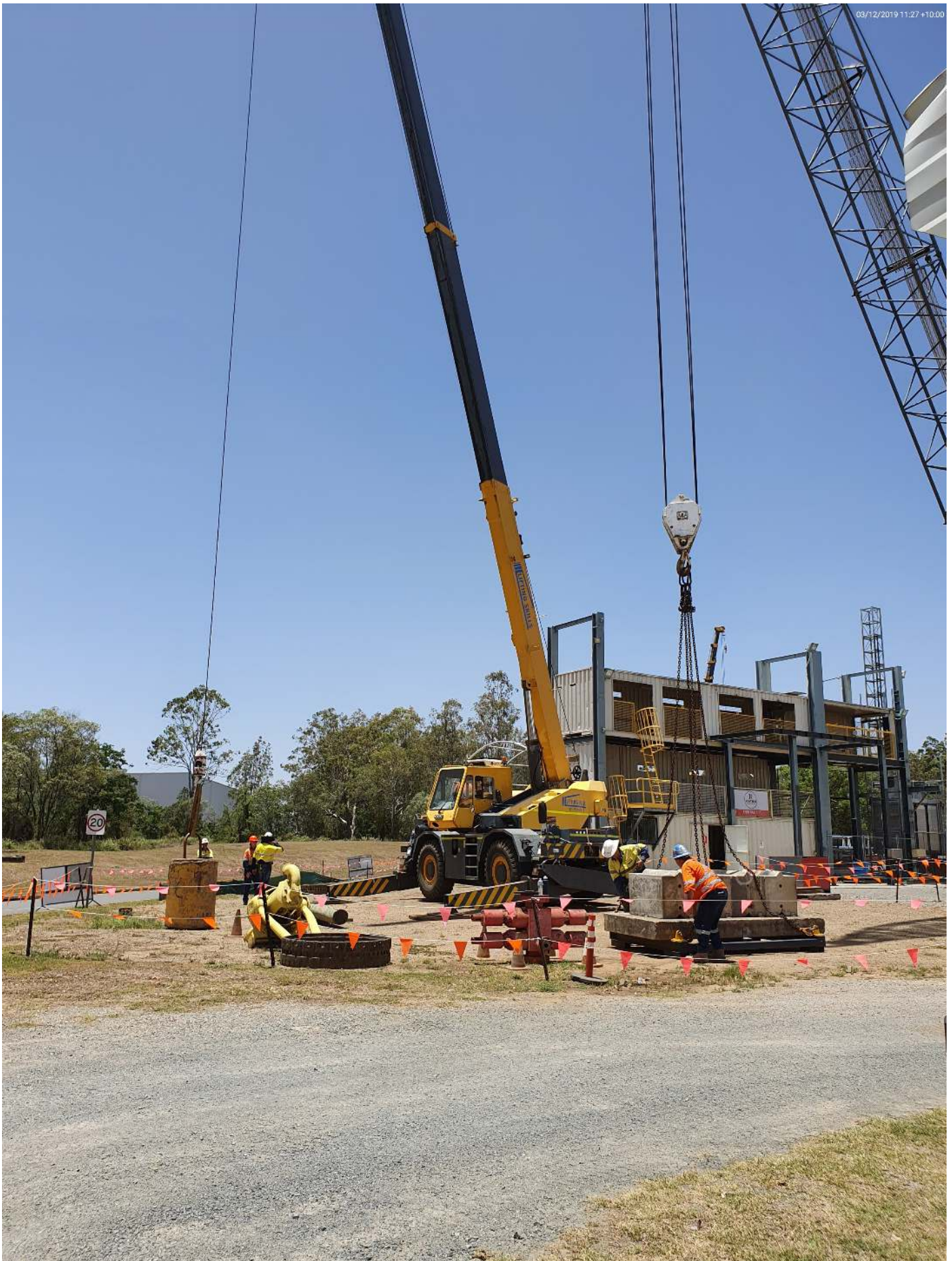
Terano crane not available, was used for training. Franna crane utilised (1 more photo)
